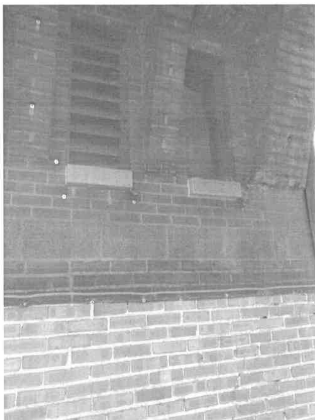
8. View of cracked and spalled brick.
