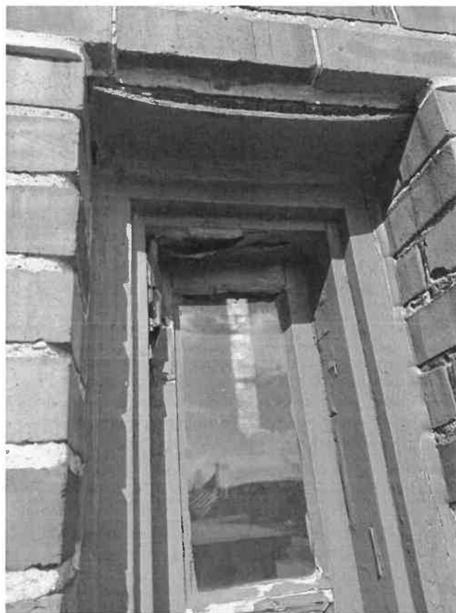
11. Window showing swelled header.
